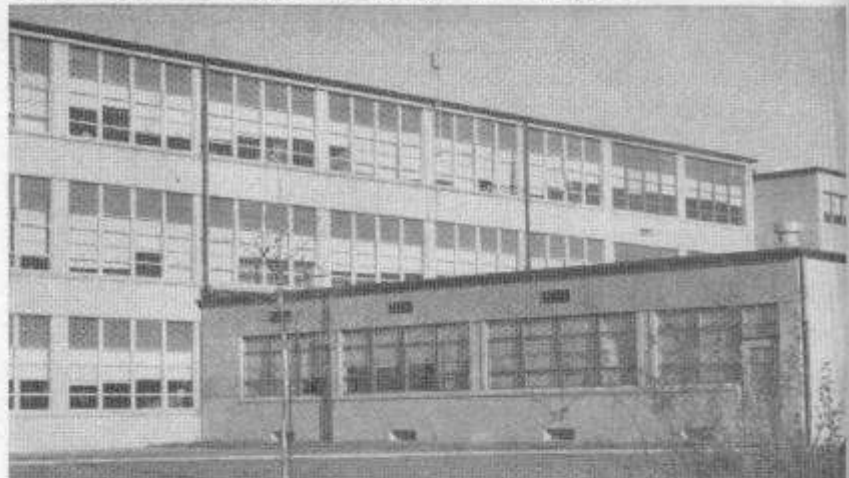
BUTLER HIGH SCHOOL, located in an area of exploding population, can almost count its years of existence by the number of additions made to it.
